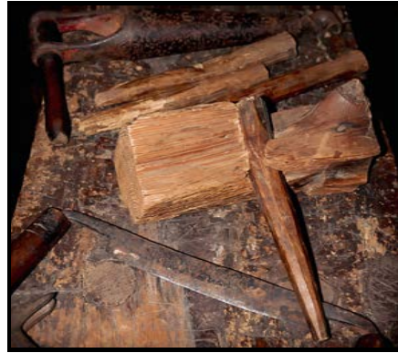
Trunnels and Beam Fragment (W14-19CBW): Four wooden pegs ("tree nails" or "trunnels") with beam remnant, taken from Nugent's Barn (cellar hole by Beaver Dam rock next to museum). 1700s.
